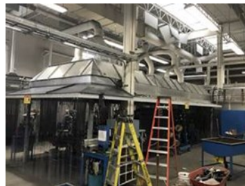
Sheet metal canopy and barriers have been installed in the Welding shop.
