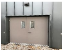
Physics pre-laboratory lab– Installed Vision glass on the exterior doors
