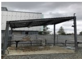
External Ceramic Gas pad branch with emergency shutoff
