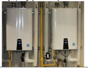
Replaced the Langley Main campus domestic hot water storage tank standby boilers that ran 24/7 to have water ready at all times, with 2 smaller condensing on demand boilers providing improved energy savings, greater demand control and reduced future maintenance costs.
