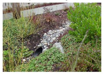
Driveway culvert for road side swale
