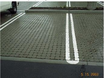
Combination of unit pavers and conventional asphalt in parking lot
