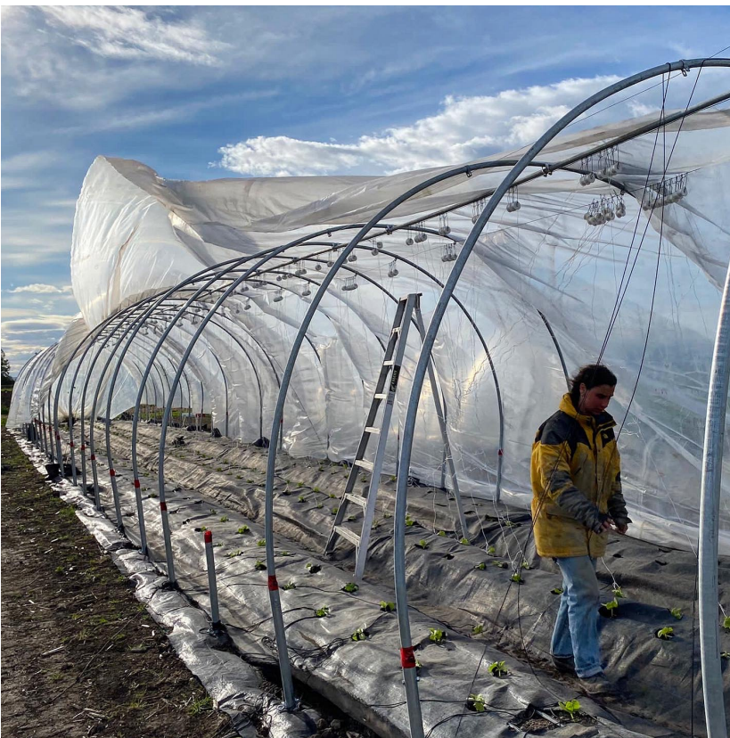
Covering the caterpillar tunnel frame with plastic sheet
