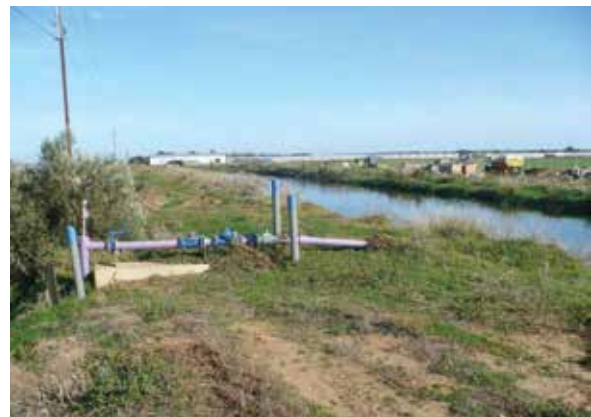
Figure 17.4. Recycled wastewater from the City of Adelaide, Australia, is pumped into an irrigation pond for a vegetable farm. Wastewater-conveying pipes are painted purple to distinguish them from freshwater conduits.
