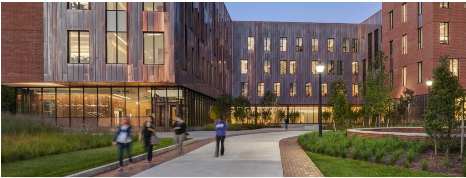
Above - Campus building that prioritizes ground-level glazing, reducing the WWR on upper levels.
