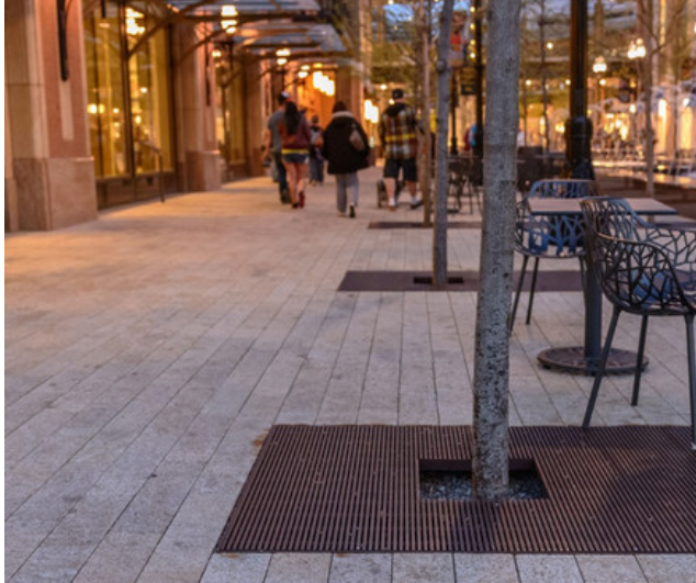
Above - Tree grates separated from the path of travel
