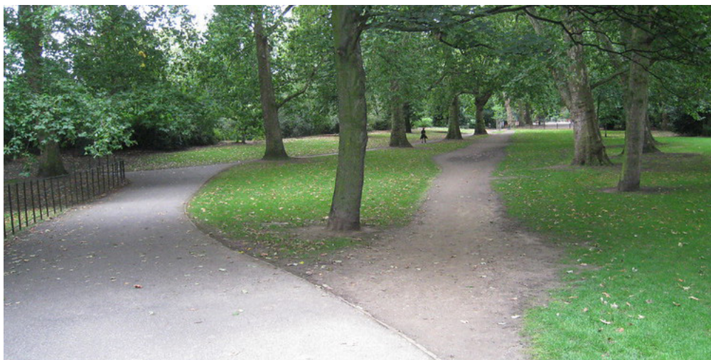
Above - Desire line deviates from the original paved path
