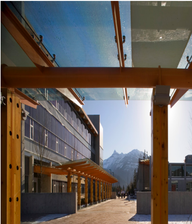
Above - Canopy of at least 3m in depth that mitigates rain and snow shedding on pedestrian paths
