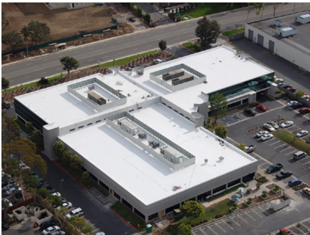
Above - High-albedo roof materials
