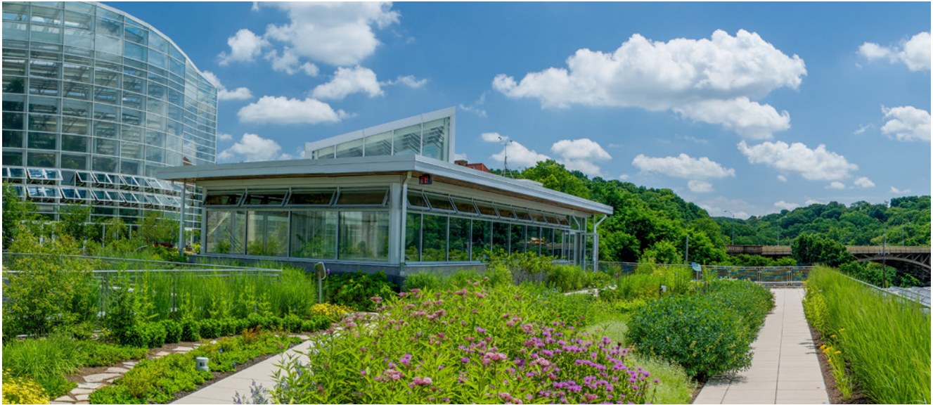
Above - Green roof designed for use
