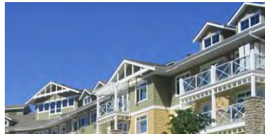
An example of varied roof forms and secondary elements such as dormers, which are used to break up a long expanse of roof.
