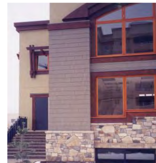
In this development, visual interest is enhanced through the use of a variety of materials, including stone detailing at the base.
