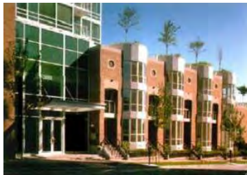
In this development, street-level row housing creates a comfortable pedestrian environment and softens the visual magnitude of the tower. The row housing provides a 3-storey podium for the tower, which is set back from the street.
