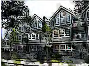
A multiple family development that creates visual interest by breaking the building mass down into volumes using both horizontal and vertical articulation.
