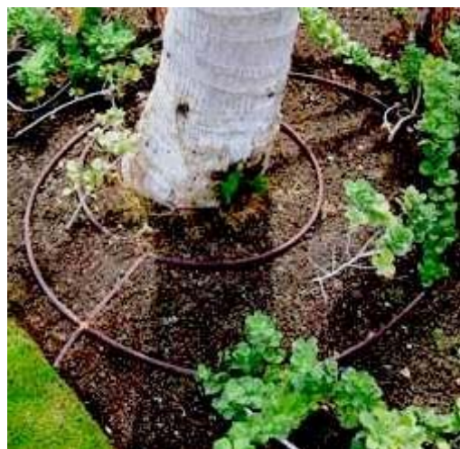
STREET TREE DRIP IRRIGATION
