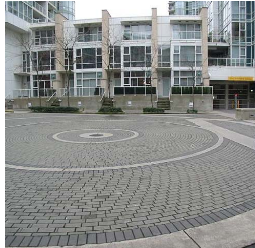
CONSOLIDATED LOADING AND PARKING
