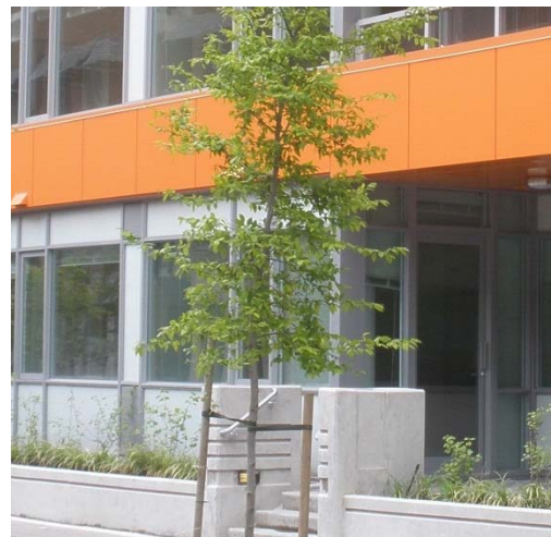
EXTERNAL TREATMENT OF PARKADE WALLS
