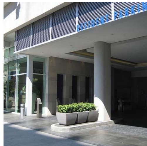
ARCHITECTURAL INTEGRATED PARKADE ENTRY
