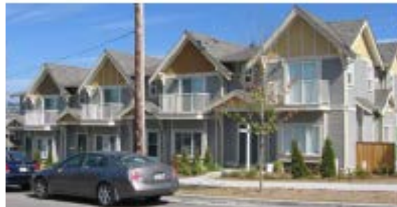
✓ Attached housing units facing the street fit within the single-family context.
