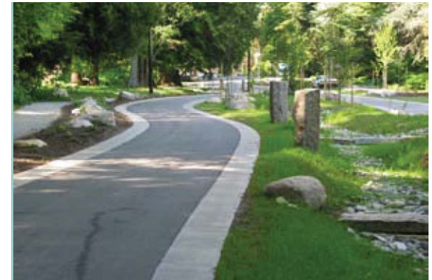
Alternative local street design provides a wide sidewalk, narrow curved traffic lanes and a constructed wetland to detain rainwater (City of Vancouver)
