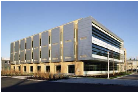
100% outdoor air is supplied to the building by trickle vents
