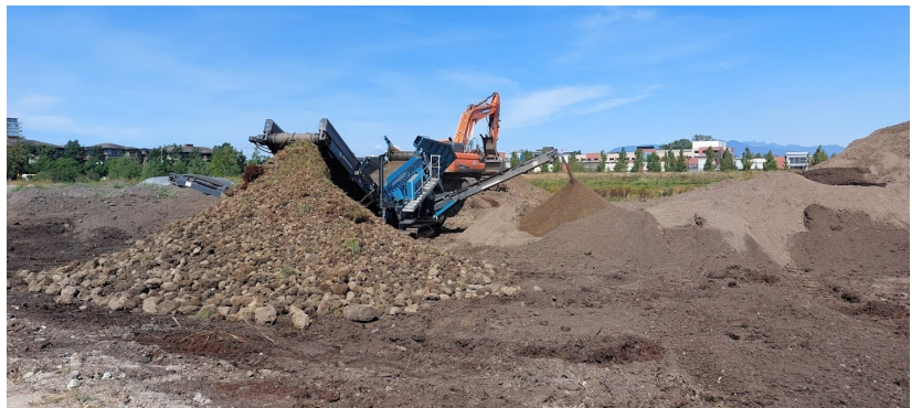
Equipment working at the site to screen the imported material prior to spreading across the site to ensure optimal quality. Sept. 2024
