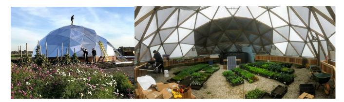
During the fall of 2018 we began the construction of our geodesic passive solar dome. This is a prefabricated kit that provides greenhouse space that can facilitate year round production without the input of fossil fuel energy. This greenhouse does not require any supplemental energy input. It captures solar radiation and relies on the design to facilitate efficient year-round heating and cooling.
