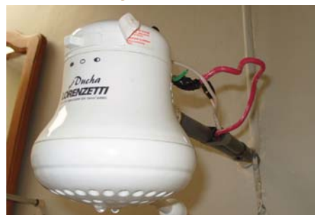
Figure 11.20 On-demand electric hot water heater. Heat is supplied to water only when needed. (credit: aviddavid, Flickr)
