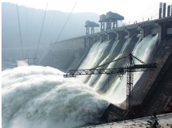
Figure 7.38 Hydroelectric facility (credit: Denis Belevich, Wikimedia Commons)
