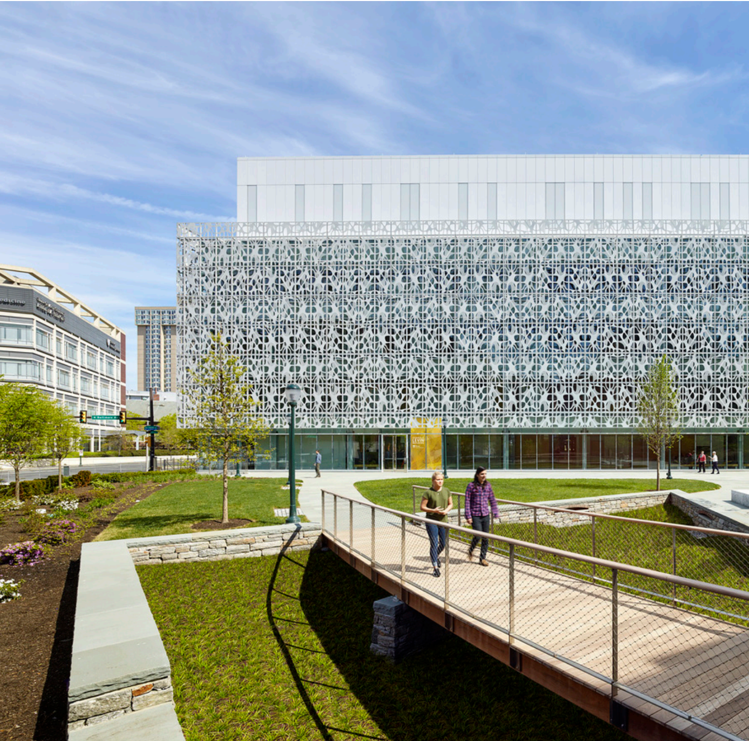
Figure 17 — Prominent landmark frontages terminate views
