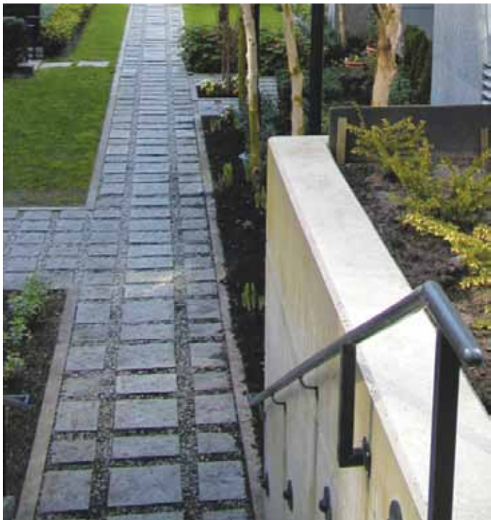
Unit pavers allow infiltration of rain water
