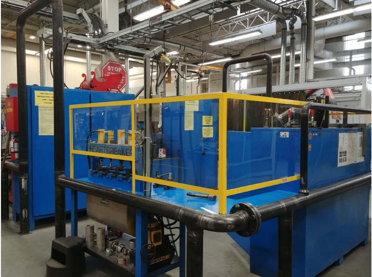
Plexiglass around CWB and instructor booth at the Welding Shop
